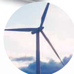
Wind power generation
